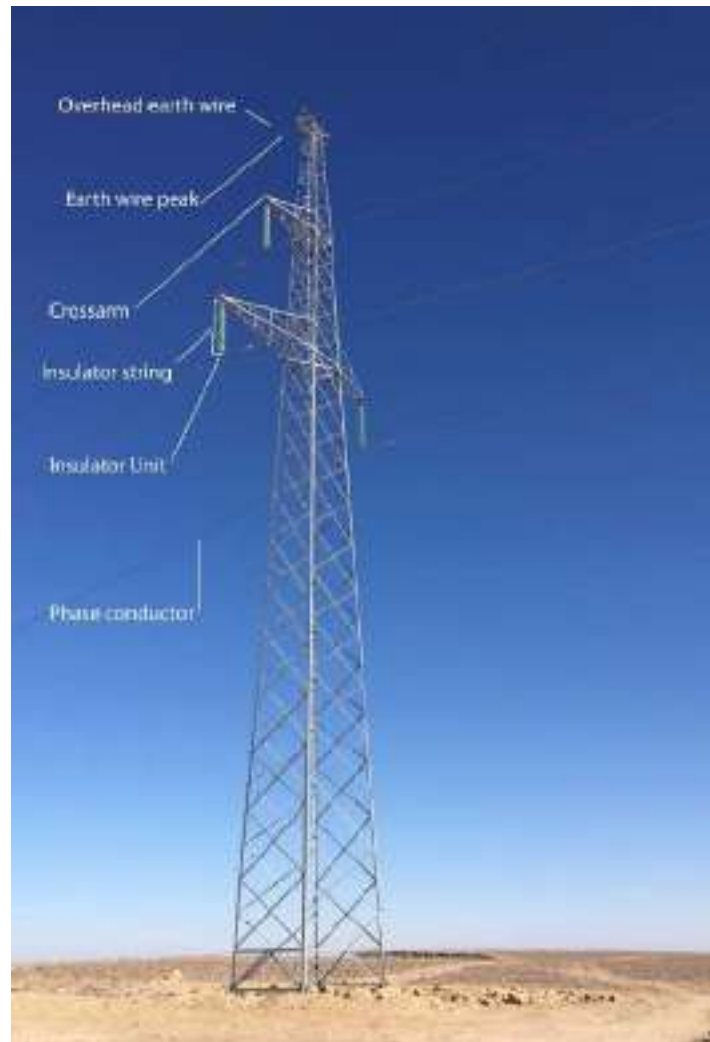
Figure 5: Components of an OHTL (Source: Juru Energy)
