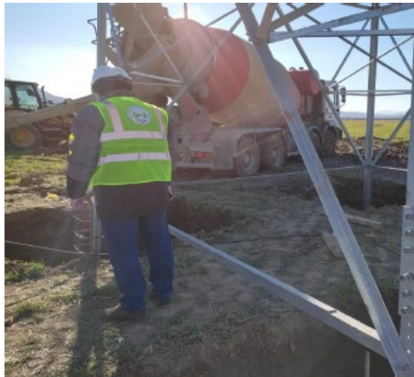
Figure 34: Example of tower foundation construction (NJDA, 2022)
