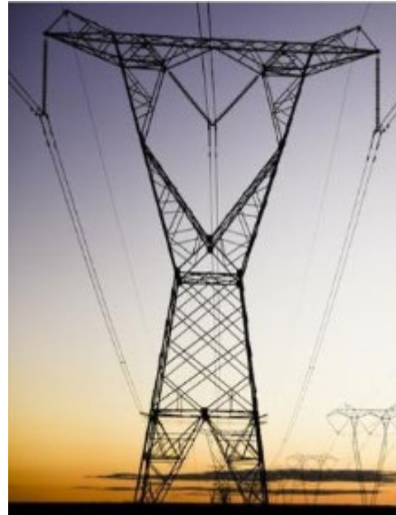
Figure 27: Self-supporting 500KV Steel Lattice Suspension Tower (single circuit) (Source: NEGU)
