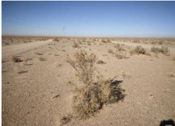
Figure 85: Existing OHTL between Kalaata and Uzunkuduk (Source: Juru Energy 2021)
