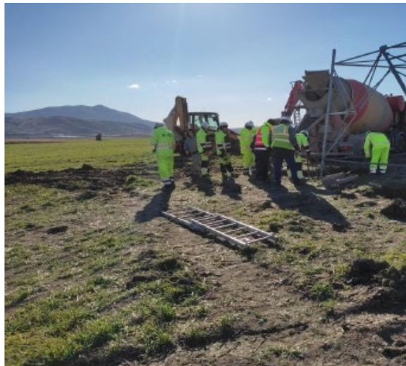
Figure 33: Example of tower foundation construction (NJDA, 2022)
