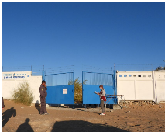
Figure 56: Water pumping station (Source: Juru Energy site visit)
