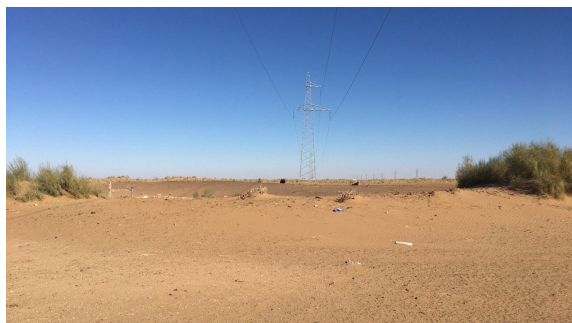
Figure 12: Existing OHTLs in the vicinity of the planned Sarimay-Dzhankeldy OHTL route (Source: Juru Energy)
