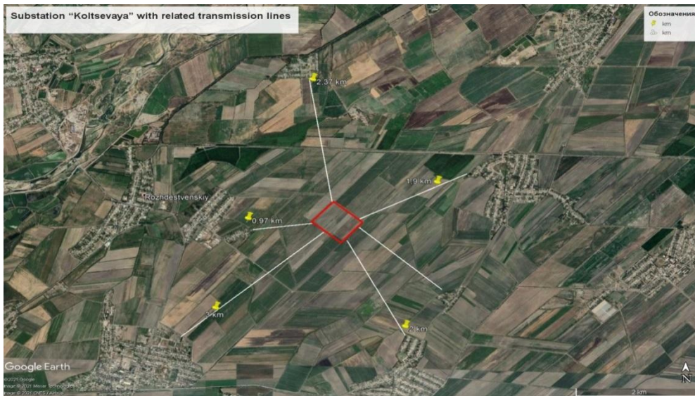
Figure 3: Substation "Koltsevaya" 500 Tashkent region
